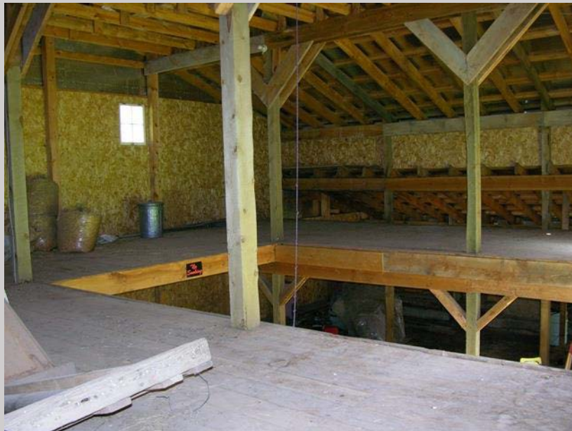
Photo 2-Interior View where modifications will make the building more useful.
